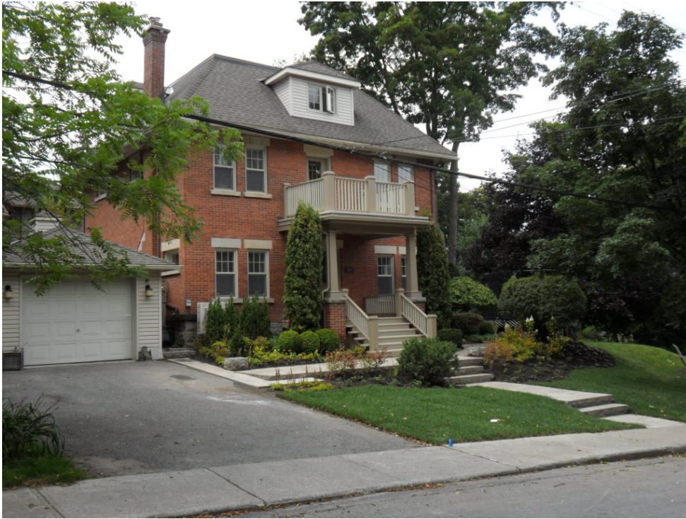
Photo no. 1 : place Irving, Ottawa, Ontario
